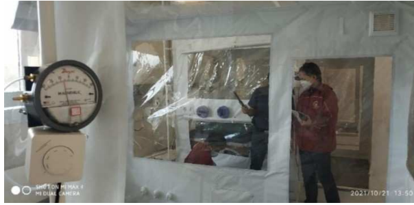
FIGURE 3. Indoor air quality assessment in isolation rooms
