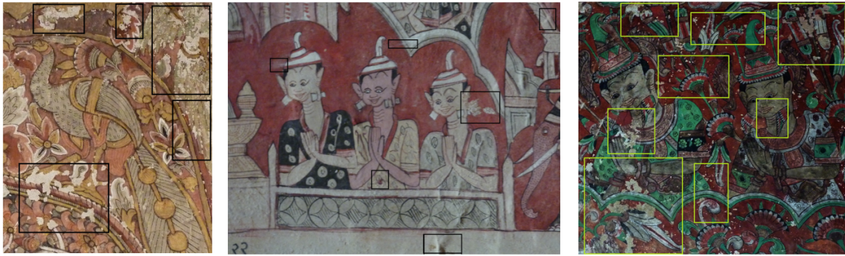
FIGURE 1. Deteriorated murals from Po-Win-Daung, Myanmar
