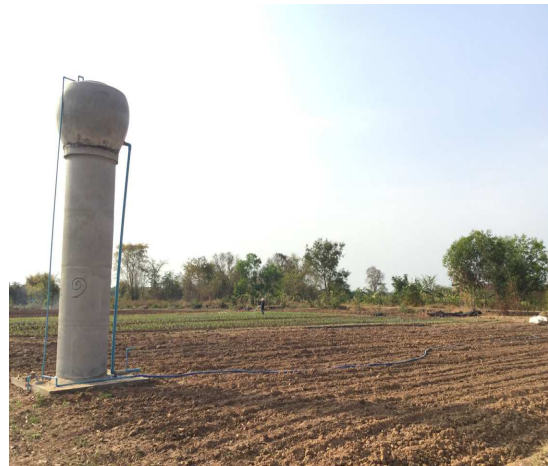
FIGURE 3. The water tank
